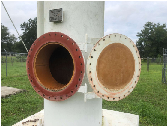
Interior base of wet riser / outlet
