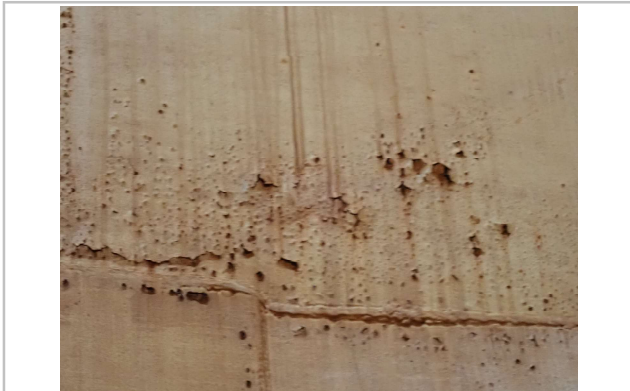
Internal walls (corrosion / d-lamination)
