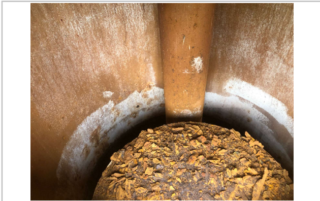
Internal walls (corrosion / d-lamination)
